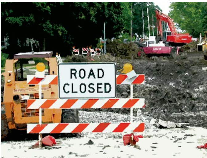
Traditional open cut pipe replacement project
